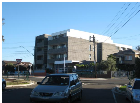
PICTURE 4 – RECENT RESIDENTIAL FLAT DEVELOPMENT – MARION STREET
